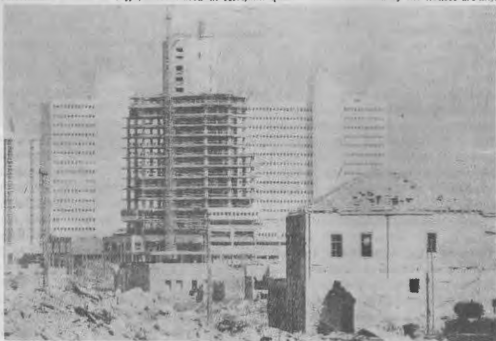
Palestinian homes deteriorate in Jaffa, while next door Tel-Aviv builds for Jews alone. About 20,000 Palestinians remain in Jaffa, concentrated in AlAjami quarter where one-third of the houses are unfit.
